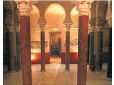
▲ Caliph al-bathes temperature room
